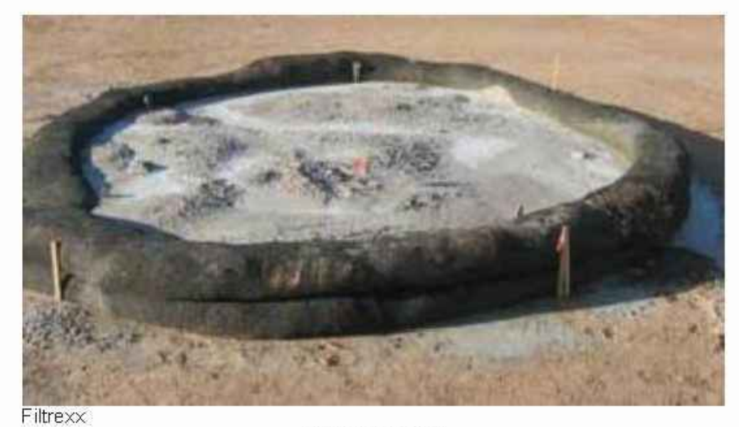
FIGURE 3.18 Typical Compost Sock Washout Installation
